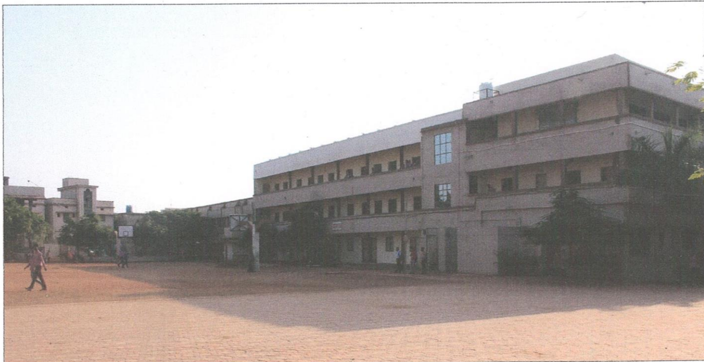
ARTS AND COMMERCE WING BUILDING
